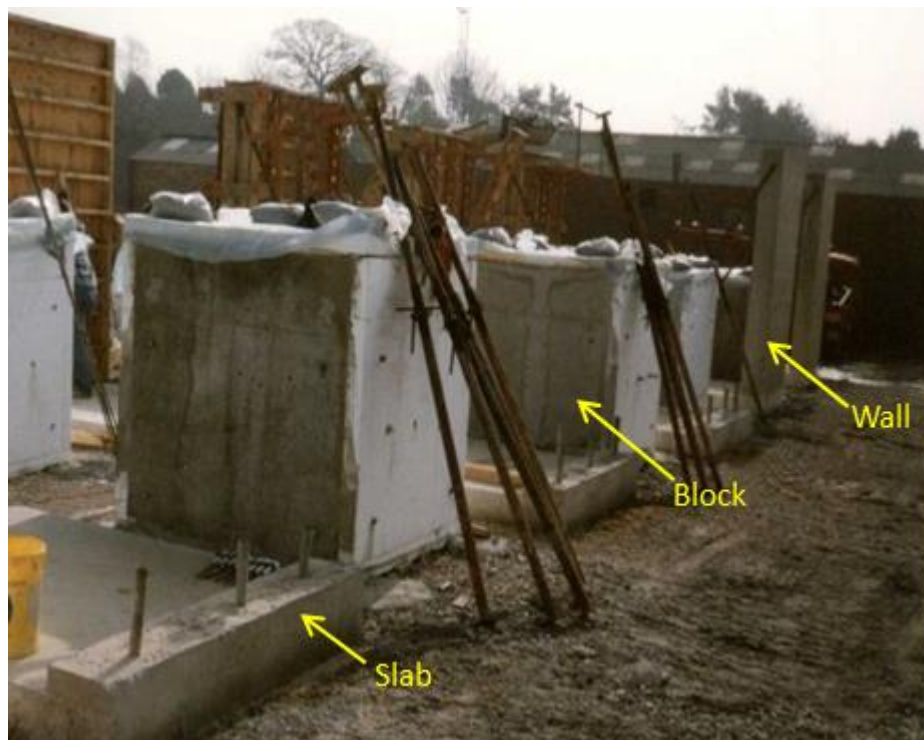
Figure 1: Structural elements used in the DTI project [2].
