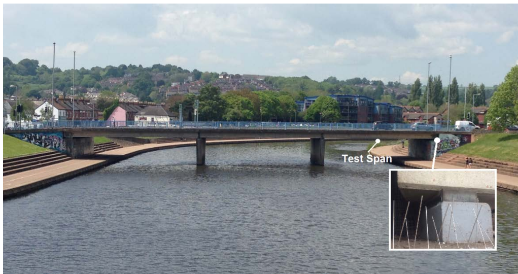
4 Fig. 2 Exe North Bridge spanning River Exe (East Elevation). The inset in the caption 5 is the photo of an elastomeric bearing at abutment location.
