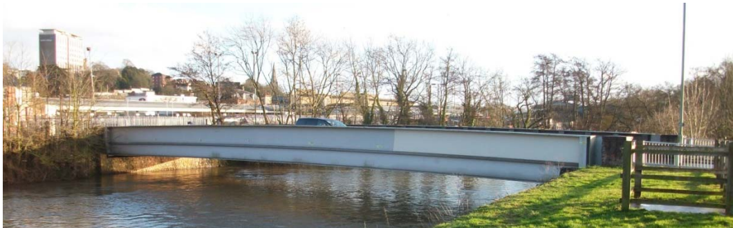
Fig. 6, Bridge used in field test.
