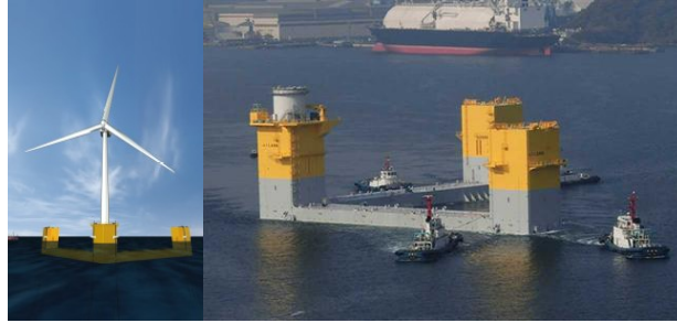
Figure 2: Braceless semisubmersible offshore wind turbine (Fukushima FORWARD [12])
