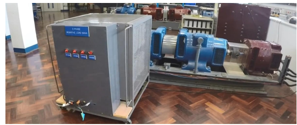
(a) Microgrid and 3-Phase Transmission Load
