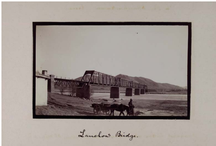
Figure 8 – Lanchow Bridge. MS15/6/11E/46.
