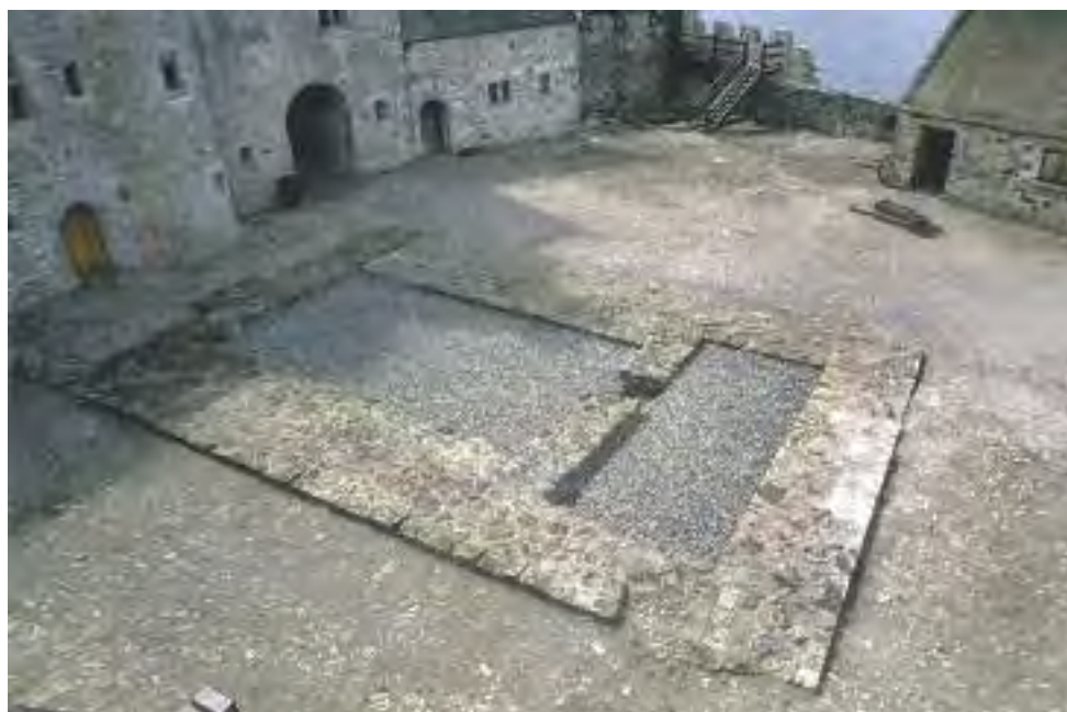
Pl. 4.9—View towards the south-west corner of the bawn interior, showing the foundations of the tower-house as displayed following completion of the conservation work (Photographic Unit, NMS).
