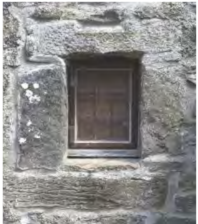
Pl. 3.13—Window in western façade of the manor house with a window-sill from an earlier building reused for the window lintel (Photographic Unit, NMS).
