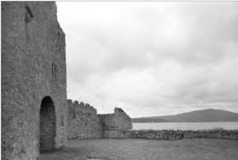
Pl. 3.30 —View of the interior of the south-east corner of the bawn, c. 1950 (Photographic Unit, NMS).
