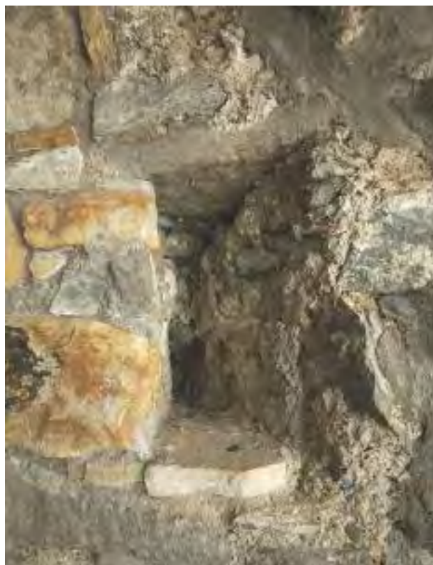
Pl. 3.25—Blocked gun loop at first-floor level within the north-west corner tower (Photographic Unit, NMS).
