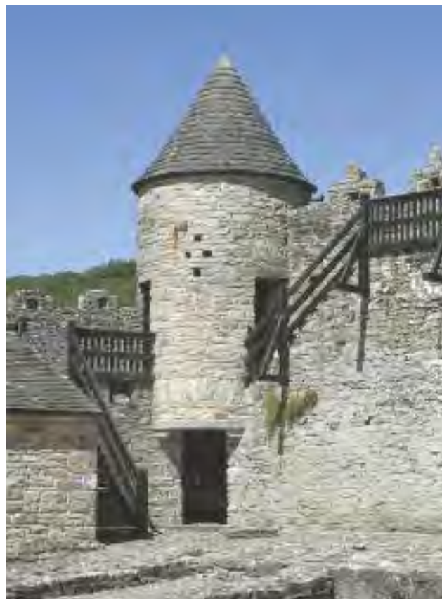
Pl. 3.20—View of restored north-west corner tower (Photographic Unit, NMS).
