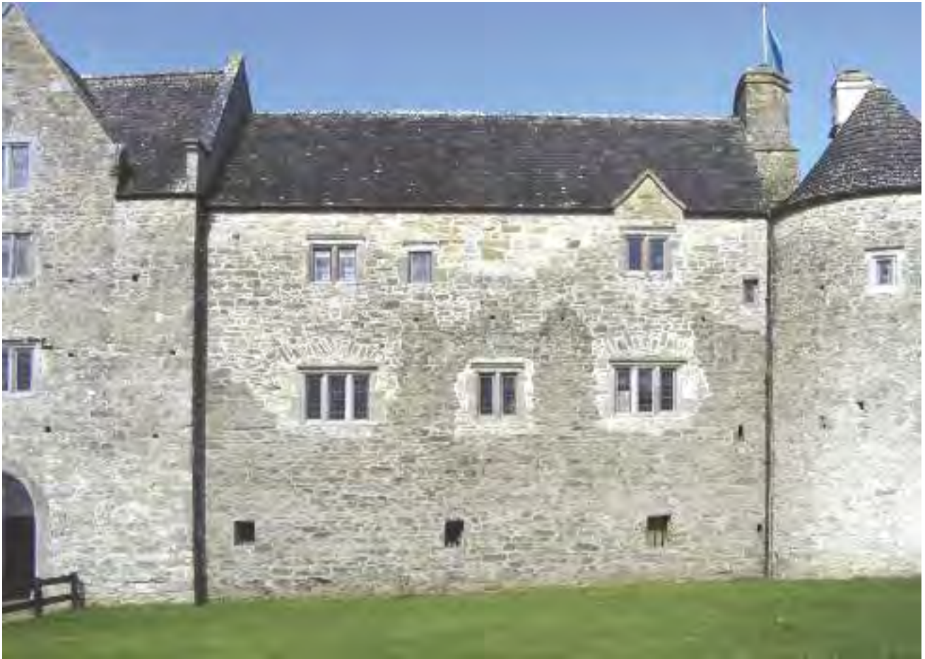
Pl. 3.14—Eastern façade of the manor house, showing evidence of the incorporation of the bawn wall into its fabric. Shading has been used to highlight the earlier bawn wall (S. Gormley).
