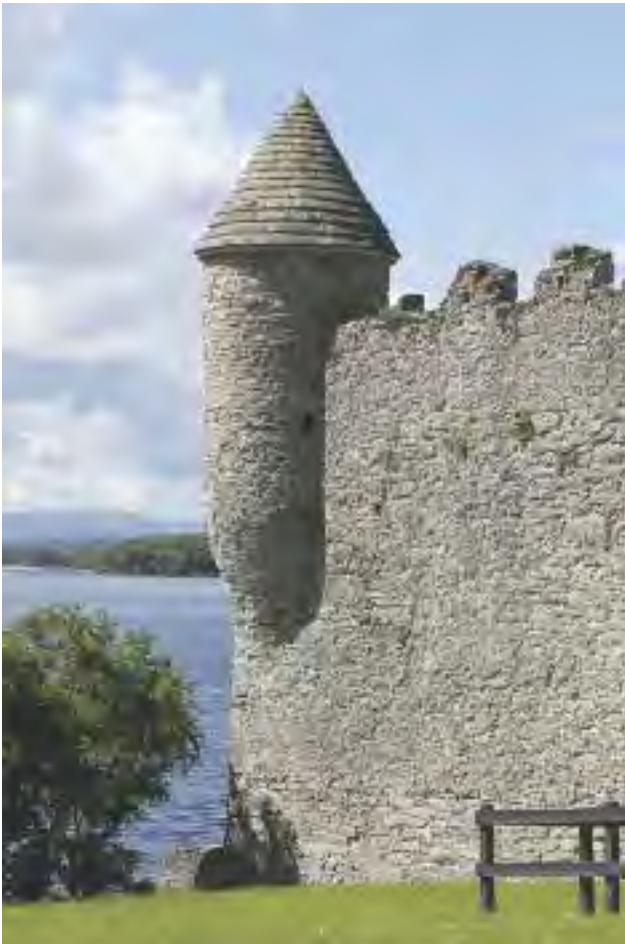
Pl. 3.31—The south-east corner turret, restored with conical roof (Photographic Unit, NMS).
