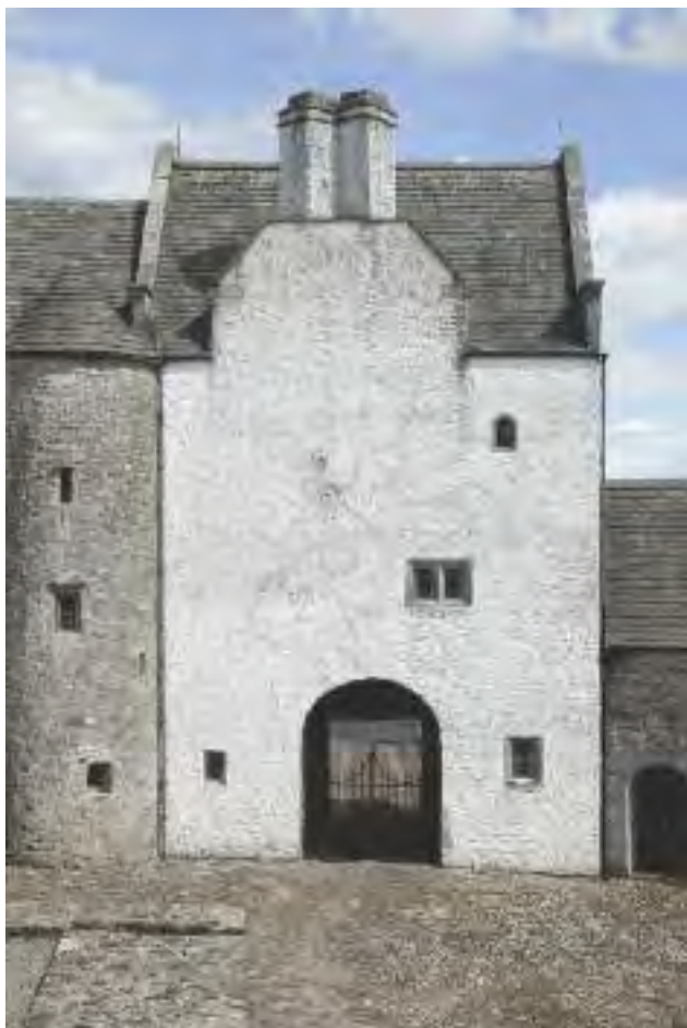
Pl. 3.9—The western façade of the gatehouse (Photographic Unit, NMS).
