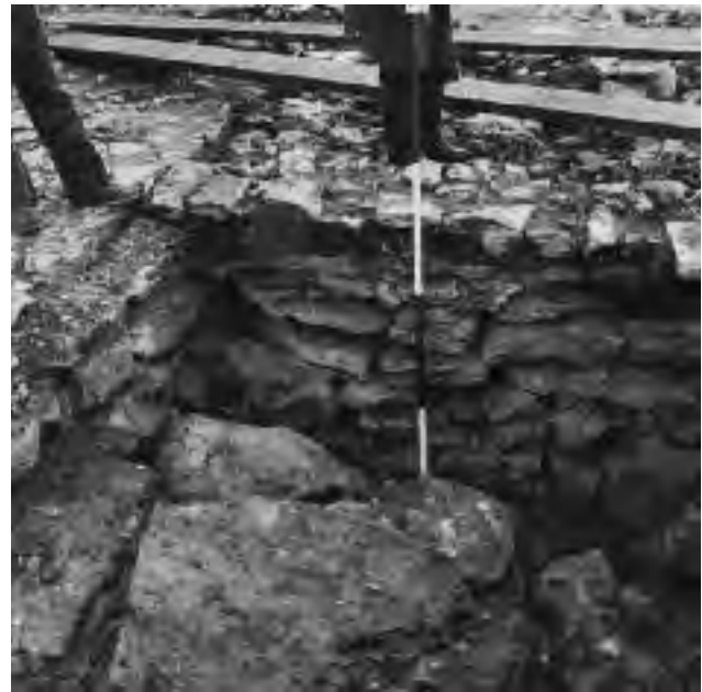
Pl. 4.14 —The north-east corner of the eastern chamber in the main chamber block, showing its abutment against the wall of the building's subsidiary chamber section (Photographic Unit, NMS).
