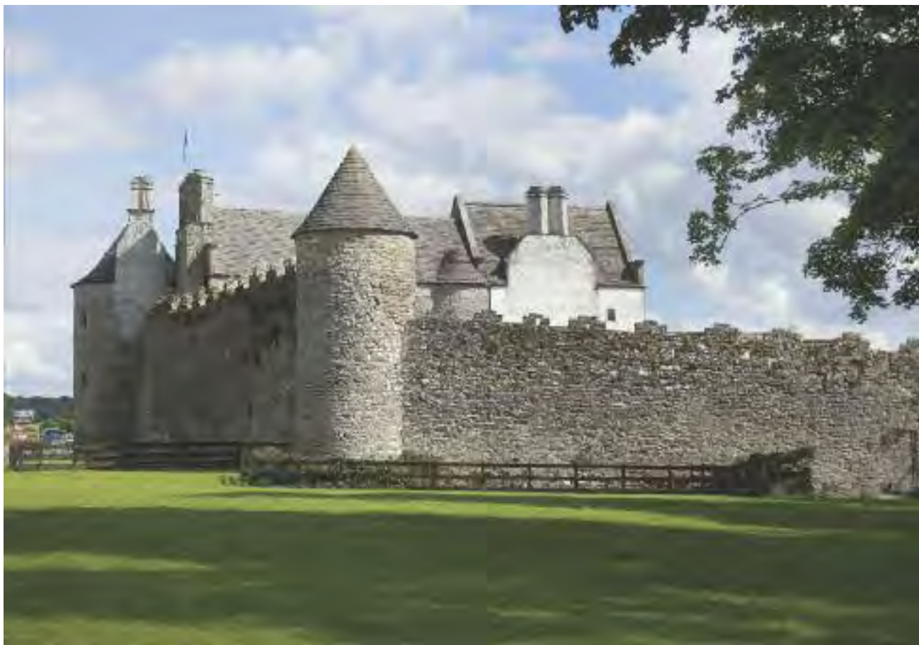
Pl. 3.24—External view of the north-west corner tower and the western bawn wall following conservation (Photographic Unit, NMS).
