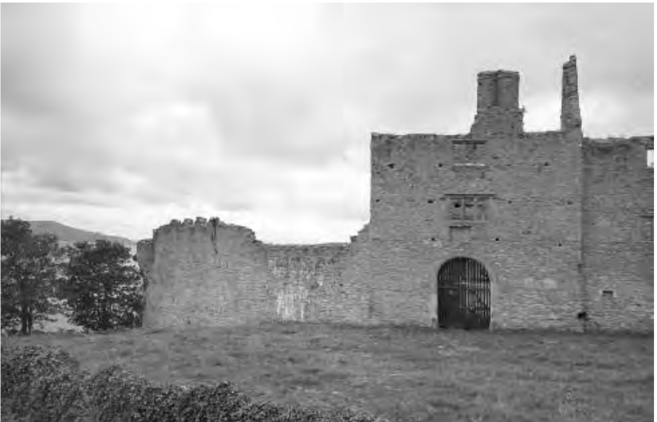
Pl. 3.6—View of the eastern façade of the gatehouse, the south-east bawn wall and the south-east turret, c. 1950 (Photographic Unit, NMS).
