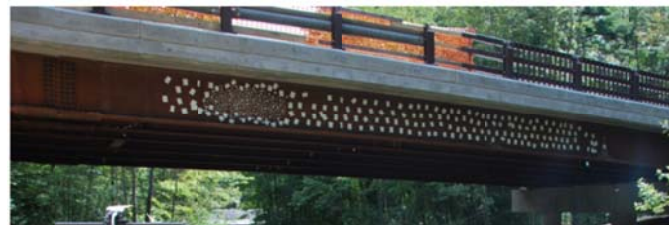
Figure 4 Speckled pattern applied for field test [16]
