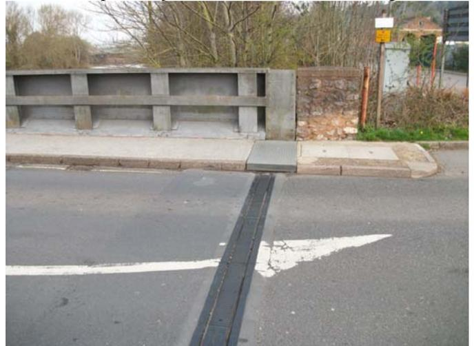
Figure 8, Deck expansion at the east end of the bridge, (this view is looking north).
