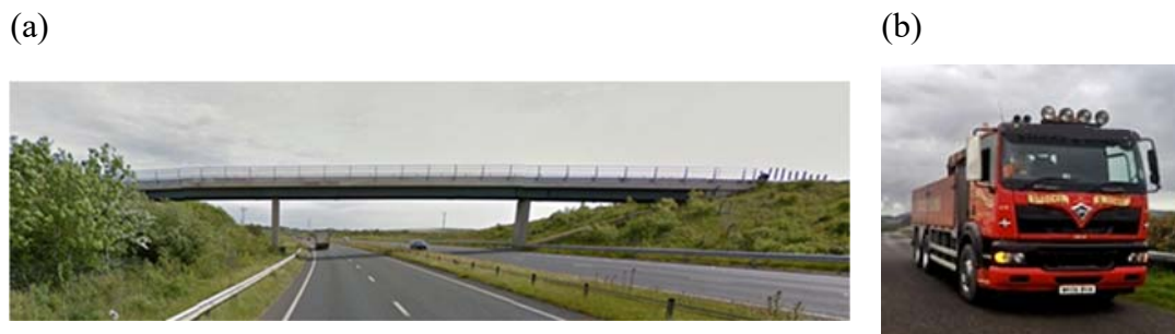
298 Fig. 3: (a) Bridge A elevation (3-span bridge); (b) Truck used in experiment
