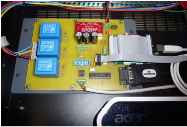
Fig. 3. Motherboard of OpenPMU system in 19" rack unit. National Instruments data acquisition board is located under larger ribbon cable. Phase estimation algorithms are computed on PC (visible in lower right corner).
