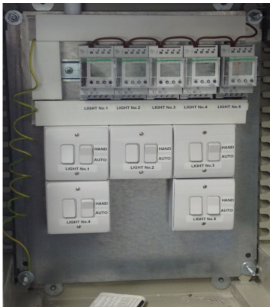
Figure 2.9. Custom made lighting unit at QUB for T5 Linda bulbs with dimmer and programmable clock system for each light unit.
