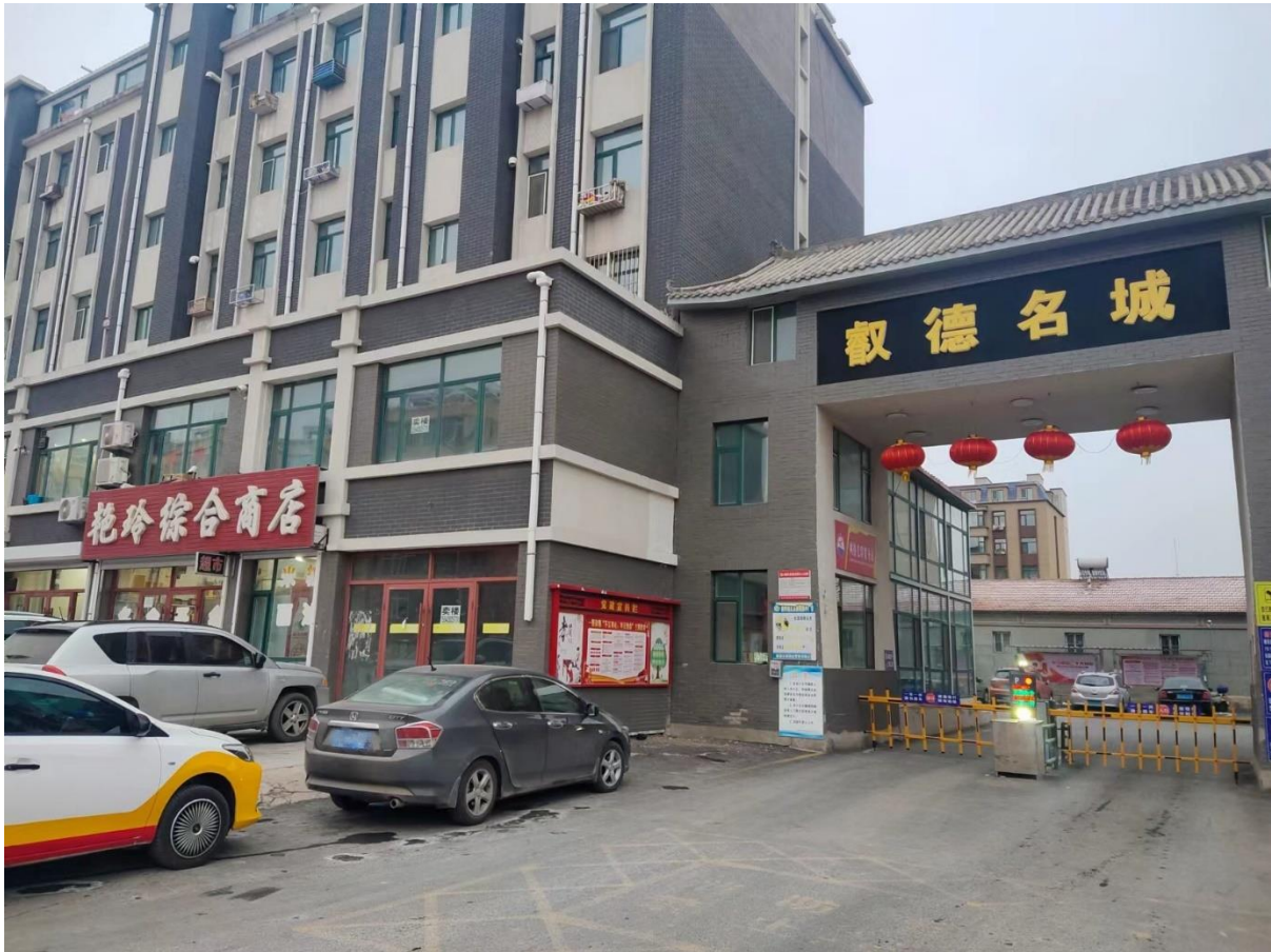
Figure 3 A Residential Compound in Taonan, Jilin Province, China (Source: author's mother's photograph taken in February 2023, permission obtained)
