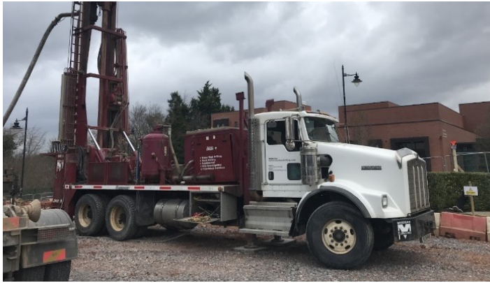
Figure 25 – Drilling operations at the new Business School
