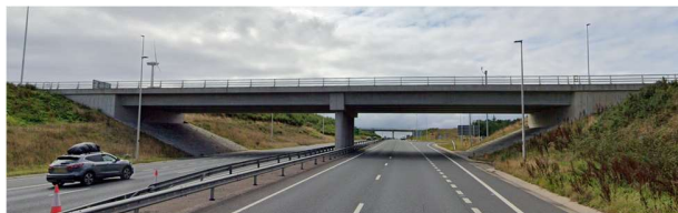
Figure 1: The beam-and-slab bridge located in N.I. used for the data collected.
